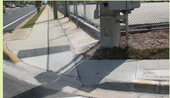
The truncated dome tactile strip is placed incorrectly within the curb ramp
