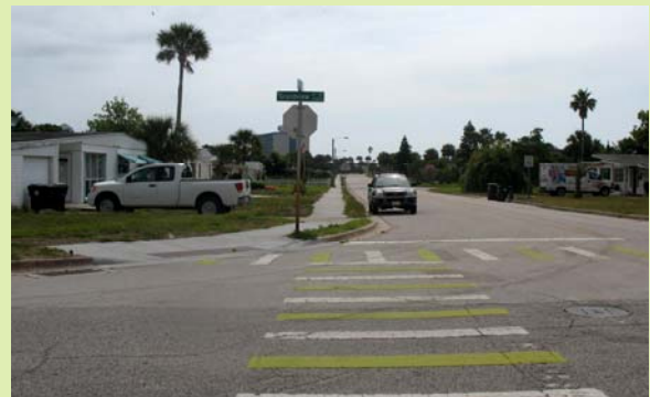
The crosswalk over Grandview Avenue does not directly connect to the curb ramp on Bel Aire Drive
