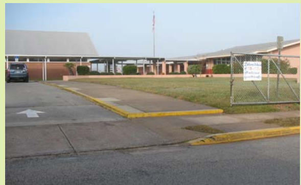
The school sidewalk does not meet the Grandview Avenue sidewalk flush to grade
