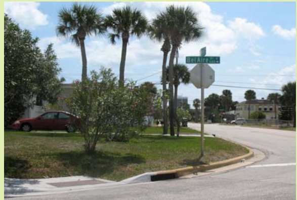
The sidewalk along Bel Aire Drive does not quite connect to the existing sidewalk on Wild Olive Avenue
