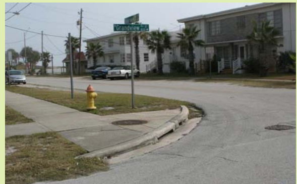
The sidewalk at the intersection of Grandview Avenue and Riverview Boulevard does not have curb ramps
